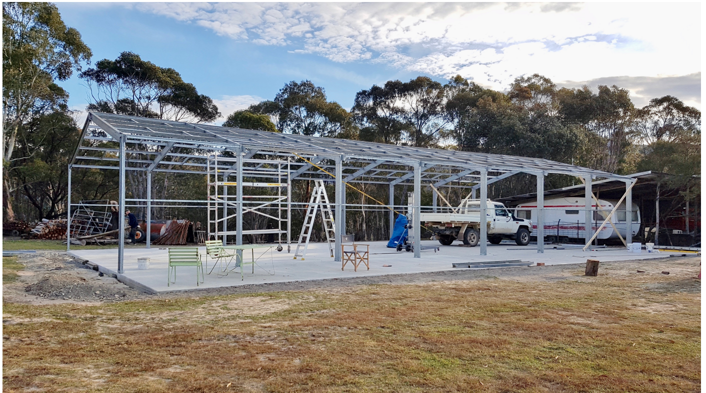
Photo 1: View of the shed frame erected 15th May, 2019. The ute was used as an anchor for straightening purposes.
